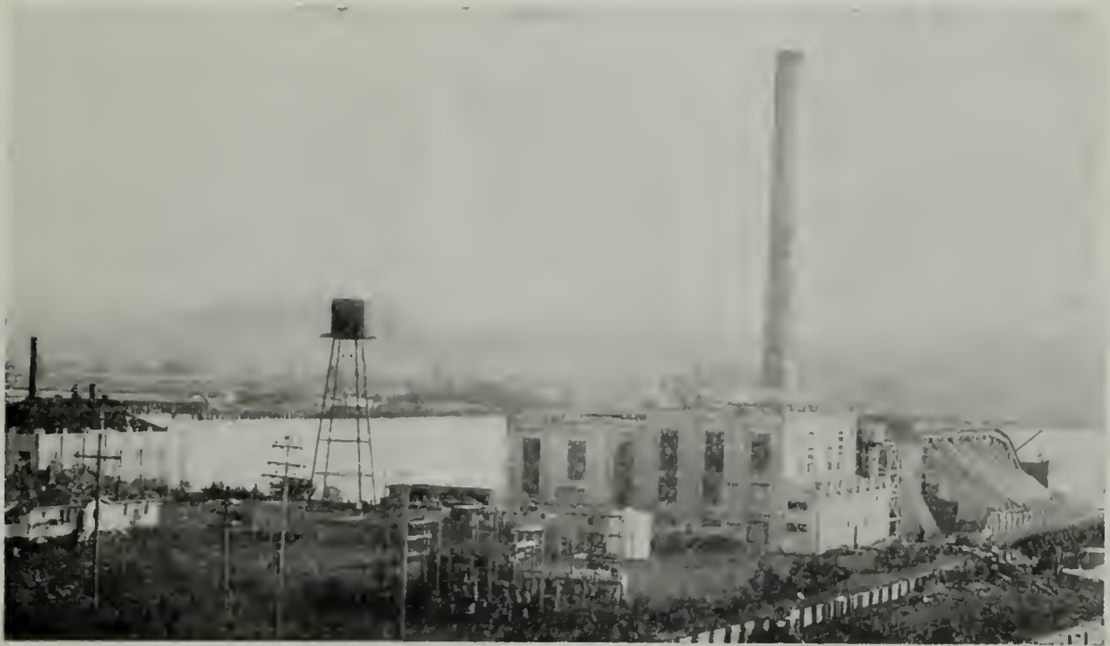
Astoria Steam Generating Station - Built in 1920 by Pacific Power & Light Company
